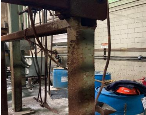
Beam on the left is near an HCL tank. The beam on the right is the same age, runs the same process but does not include an HCL tank. HCL is very corrosive to equipment.
